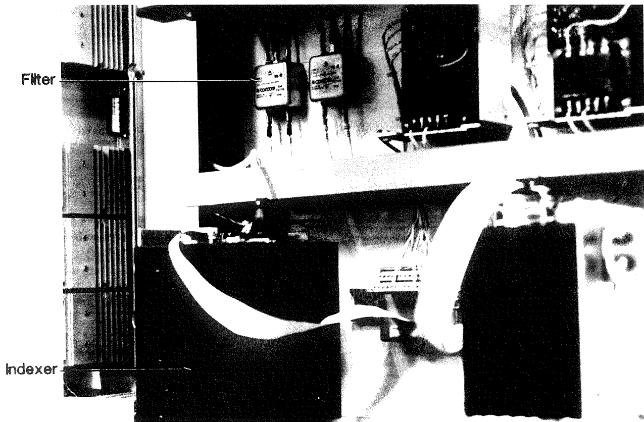
FIGURE 2 Filter Mounted Adjacent To Indexer
